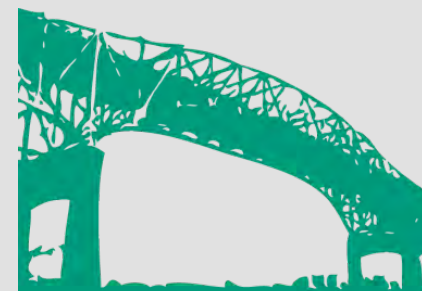
I-10 LAKE CHARLES CALCASIEU RIVER BRIDGE
